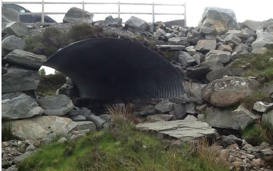
Plate 4: Existing access track and arched culvert over Allt Ghuibais Mor
