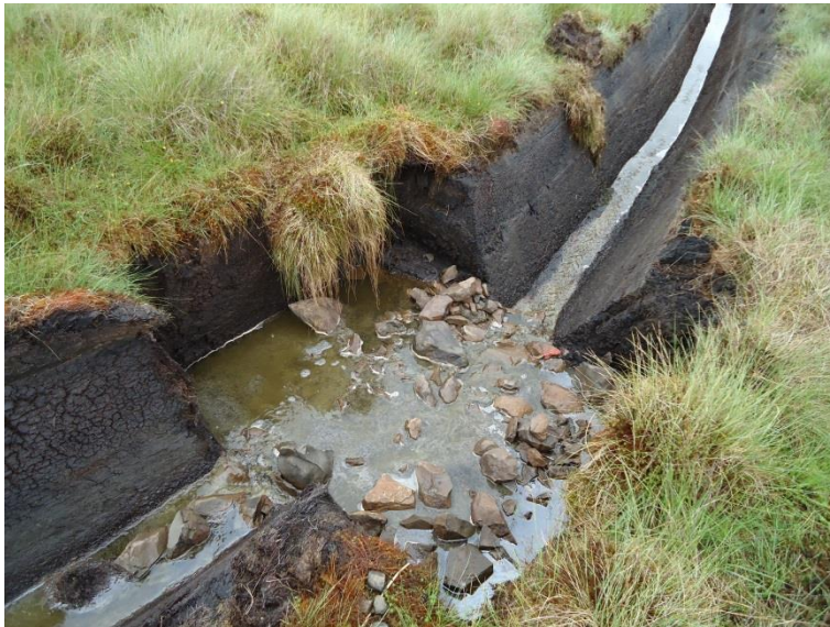
Plate 2: Typical silt trap
